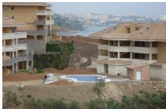
Construction site (Malaga, Spain). Credits: M. Palacios
