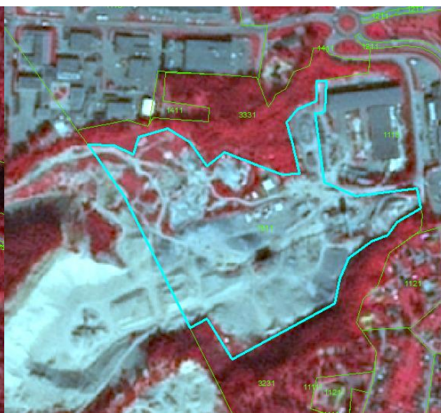
Delineation of construction site at Skien (Norway). SPOT-5 (2.5m) (1/2/3 Band Combination). Date: 2010-08-11. Source: CNES 2011©, Distribution Airbus DS/Spot Image
