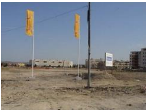
Construction site (Cadiz, Spain). Credits: M. Palacios
