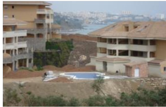
Construction site (Malaga, Spain). Credits: M. Palacios.
