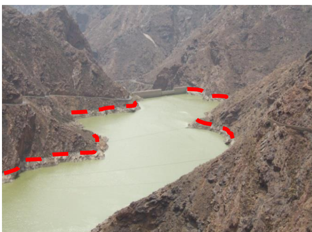
Delimitation of reservoirs using the maximum water lever. This is the wrong interpretation . Reservoir in Canary Island (Spain). Credit: M. Palacios.
