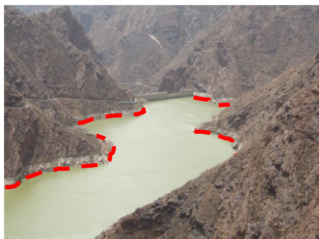
Delimitation of reservoirs using the current water level. This is the correct interpretation . Reservoir in Canary Island (Spain). Credit: M. Palacios.
