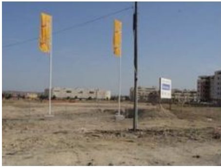
Construction site (Cadiz, Spain). Credits: M. Palacios.
